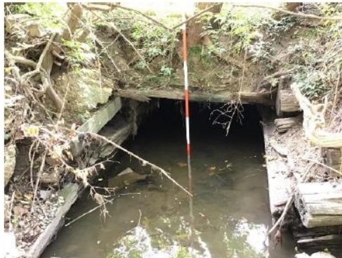
Figure 7: BA00013 Failing Timber at Outfall Section
